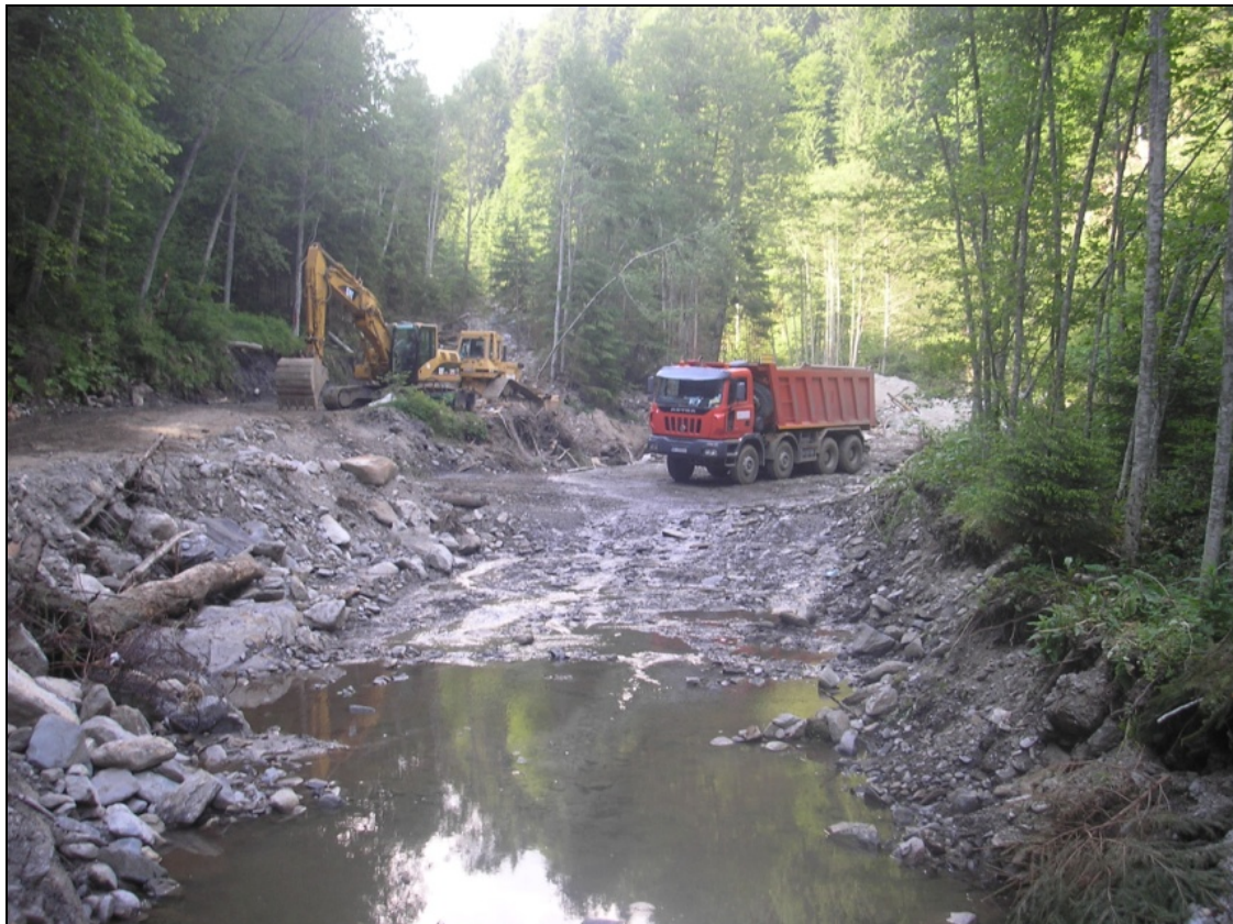
Figure 1: Heavy construction equipment work in the Capra Stream.
