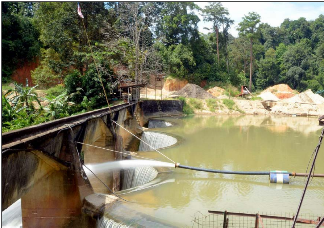
Figure 7: Water intake of Pong Dam, Perak, Malaysia.
