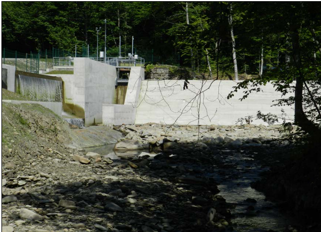
Figure 2: Tur'ya-Polianska small hydropower plant.
