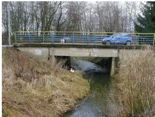
Figure 4: The concrete bridge before strengthening
