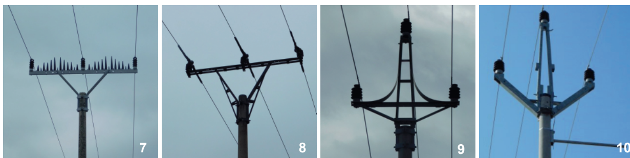
Fig. 7–11. Correctly installed and undamaged components used as mitigation measures on basic cross-arms: racks (7) or plastic covers (on horizontal cross-arms and upright insulators; 8), plastic strips (on Delta cross-arm; 9) or simple perch (used with Pařát, 10, and Delta variant cross-arms, 11).
