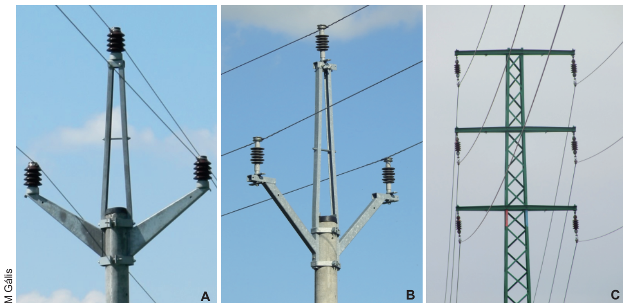
Fig. 12. Effective solutions for protecting birds from electrocution: Antibird (A), Ecobird (B) consoles and suspension pylon with hanging jumper wires (C).
