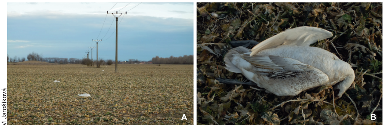
Fig. 15. Carcasses of mute swans in an oil-seed rape field used as foraging habitat, crossed by 22 kV power line (A) and visible burn marks on feathers (B) after collision-electrocution.
