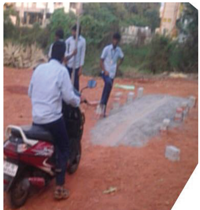
Fig. 6 Passage of a scooter along the central section of the unpaved road
