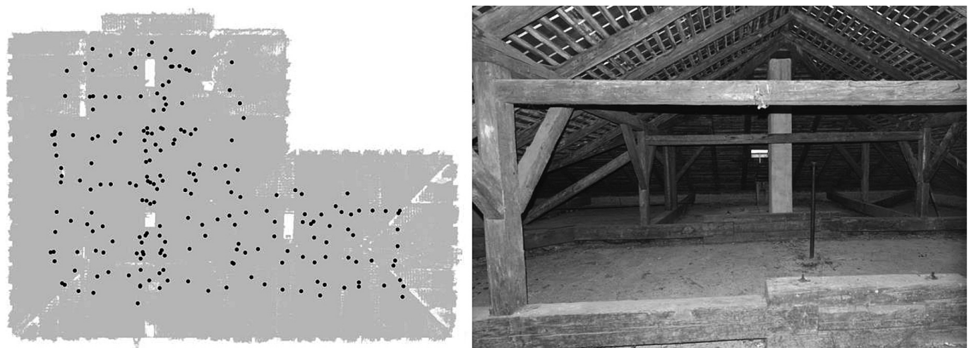
Fig. 3 Camera positions inside the truss structure (left) and an image taken by the DSLR camera (right).
