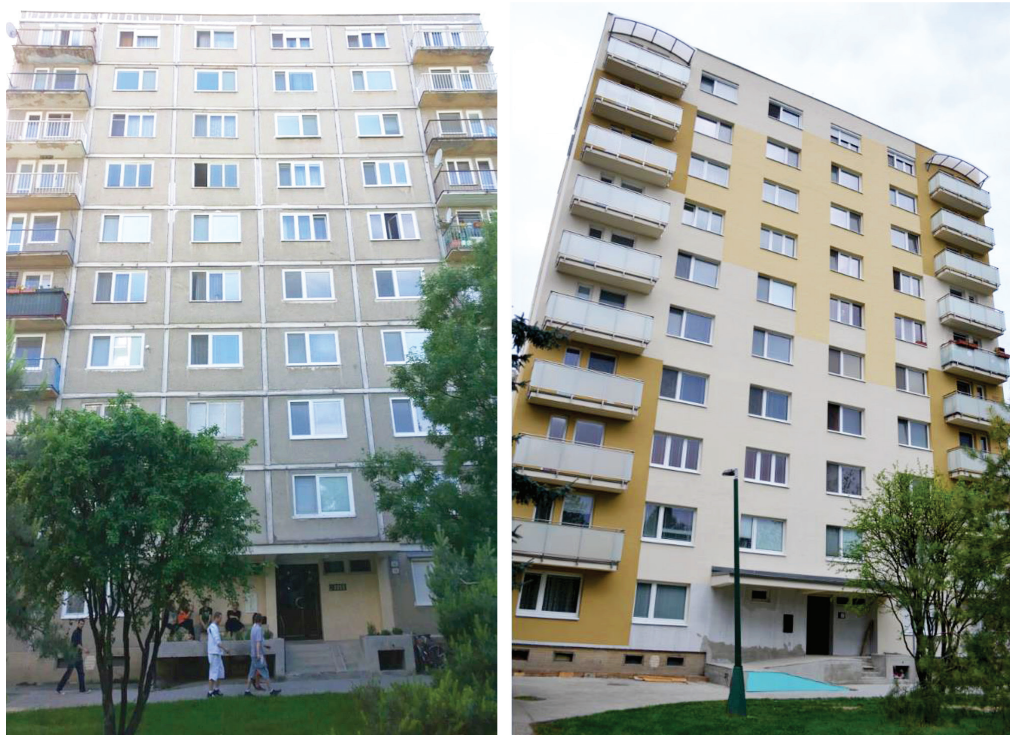
Fig. 1 The evaluated dwelling before and after the refurbishment.
