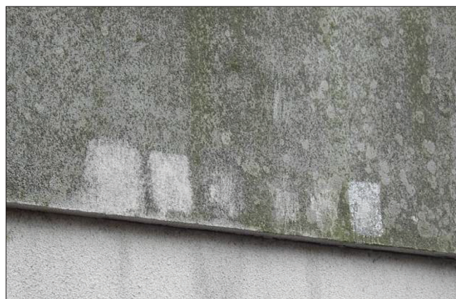
Fig. 2 Records of decontamination experiment on ETICS in 2006. Noted increase of new microorganisms, e.g., in Square No. 6 (from the left). Sample No. 1- destruction of microorganisms outside the designated area (Antošová, N., 2007).
