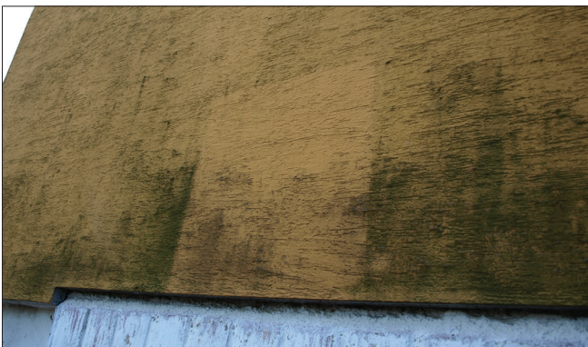
Fig. 6 Records of the decontamination experiment on ETICS. State of the sample in January 2012; this sample was not washed with water after the application of a biocide. (Picture from the archives of the author's experiment)
