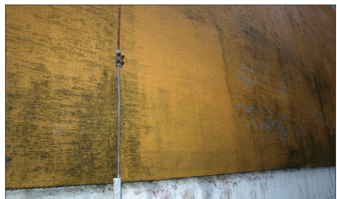
Fig. 9 Records of the decontamination experiment on the ETICS. State of the washed sample from Fig. 7, now in January 2013. (Picture from the archives of the author's experiment).
