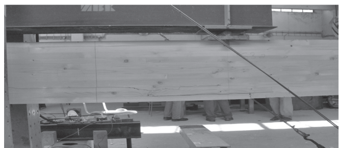
Fig. 5: First cracks of the beam (Beam №3)
