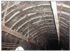
Fig. 2. Support of the bottom gate K-2: (a) support with mechanical lining, (b) support with traditional lining
