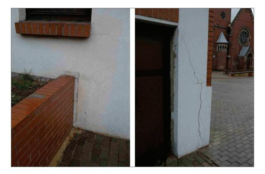
Fig. 12. Displacement of the building illustrated by original location of retaining wall
