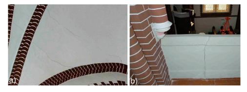
Fig. 11. Damage sustained by the church: (a) cracks in vault above main nave, (b) cracks in choir loft
