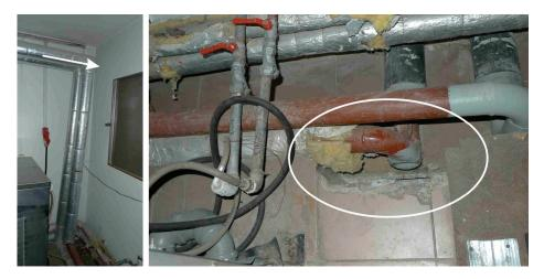
Fig. 17. NH laundry room. Visibly bent pipes and incuts made to protect the piping from damage
