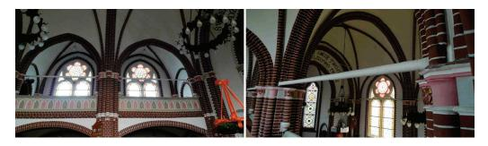
Fig. 4. Steel tie-beams protecting against mining damage
