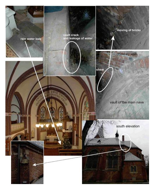
Fig. 10. Damaged vaults and crosswall of the church
