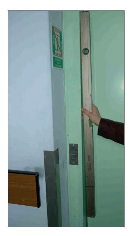
Fig. 14. Vertical tilt of lift shaft
