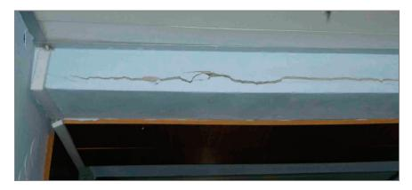
Fig. 15. Crack in places of dilation between building's segments
