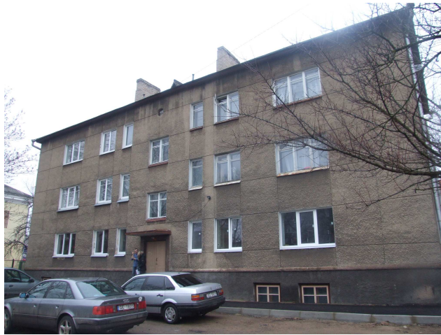
Fig. 1. Reference building: typical three-storey residential building in Latvia (built in 1960s)
