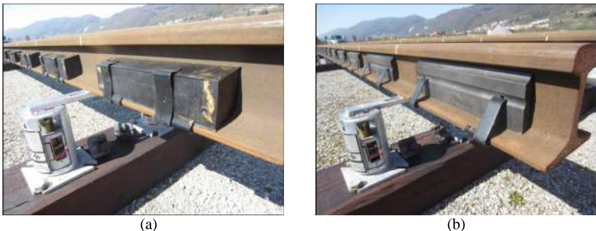
Figure 1. Rail dampers: (a) TATA Steel; (b) Vossloh [6].
