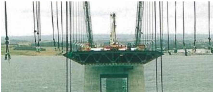
Figure 8. Storebaelt Bridge deck (1998), depth ~ 4.5 m, self weight ~ 0.35 t/m 2
