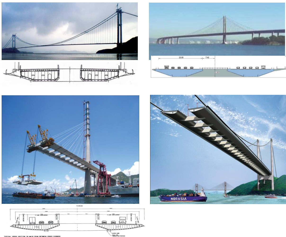
Figure 14. Clockwise: Xihoumen Bridge (China 2009), New Oakland Bridge (USA, 2013), Tsing Lung Bridge (Hong Kong, design), Stonecutters Bridge (Hong Kong, 2009).
