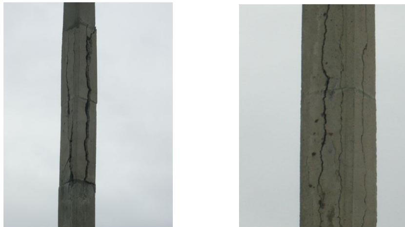
**Figure 2.** Cracks at some of the bridge concrete hangers
