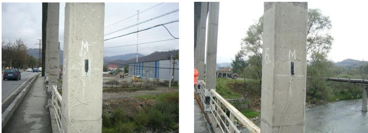
**Figure 4.** Electro-resistive transducers placed on the concrete hangers
