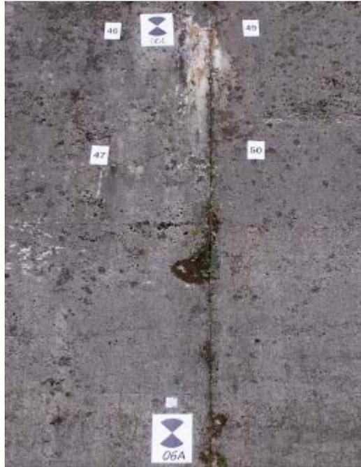
**Fig. 6.** Used survey targets on the concrete surface.
