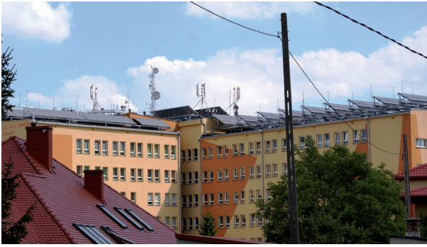
Photo 3. Independent Public Health-Care Centre at Radzyń Podlaski (Lublin voivodeship). An example of a TI project co-funded by the ROPV (2007–2013) in a town of up to 20,000 population.
