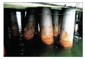
*Fig. 6. Sea corrosion of piles [10]*
