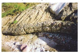
Fig. 3. Gabions composing the seawall in the region of "Bałtyk", damaged in 1998 (photo courtesy of W. Subotowicz)
