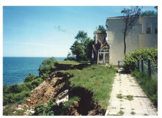
Fig. 2. The leisure centre "Horyzont" situated on the edge of an active cliff and damaged in 2002.
