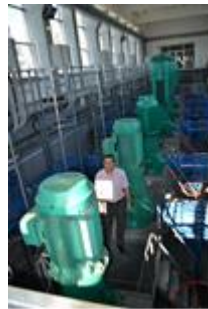
Photo 2. The “CITY” pumping plant
