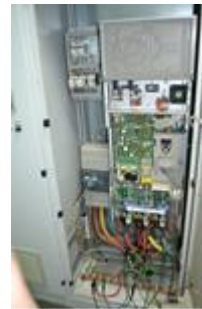
Photo 3. The static frequency converter
