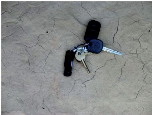
Figure 1. Plastic shrinkage cracking of concrete [1].
