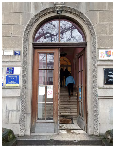
Figure 4. The entrance door of Secondary School, Bosa Milićević
