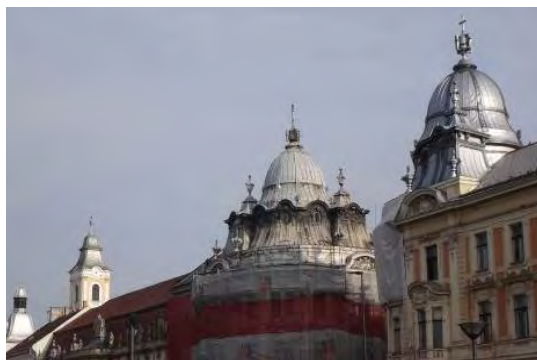
Figure 2. Domes covered with galvanized sheets on the main square of Cluj-Napoca
