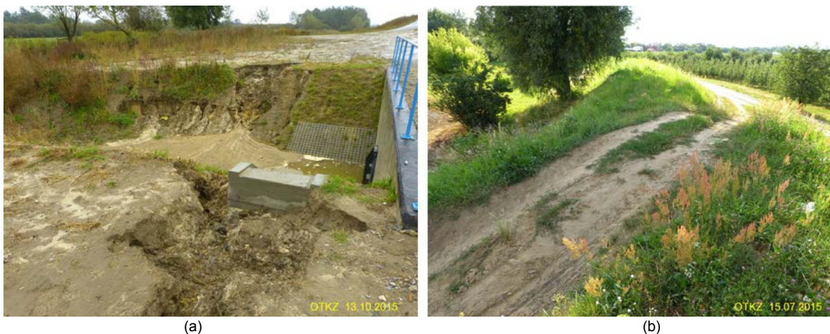
Figure 2. Presents an example of a landslide in Poland in 2015 and levee surface damage caused by people. Photo by Janusz Orzepowski
