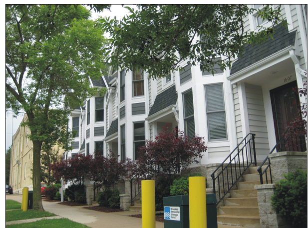
Fig. 3: Photo of a residential brownfield redevelopment project (Photo: Brendon Jones)
