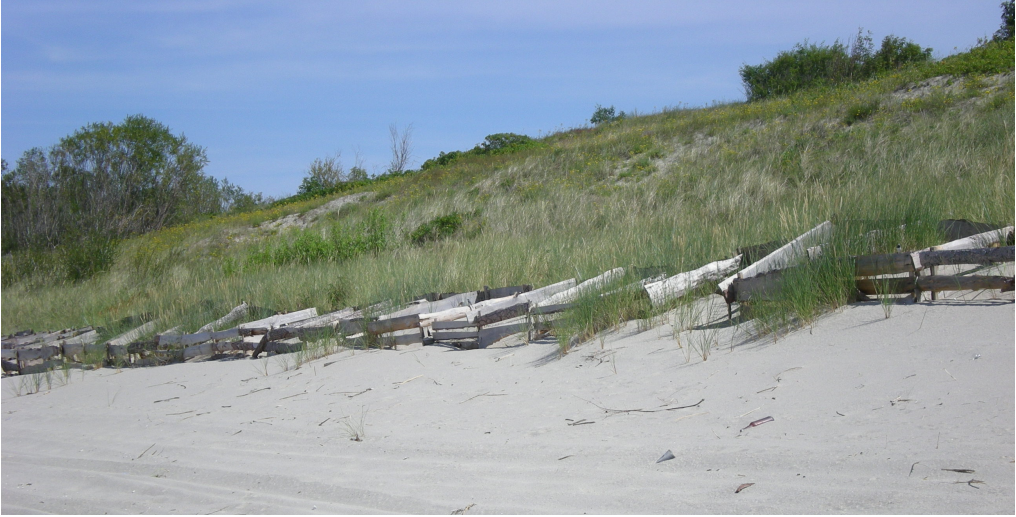
Fig. 3. Light wooden sand-accumulation structures built at the dune toe in the Russian coastal segment of the Vistula Spit in 1976
