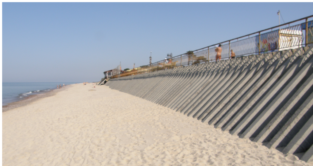
Fig. 11. A massive permeable revetment with pavement on top in Lesnoy, built in 1995
