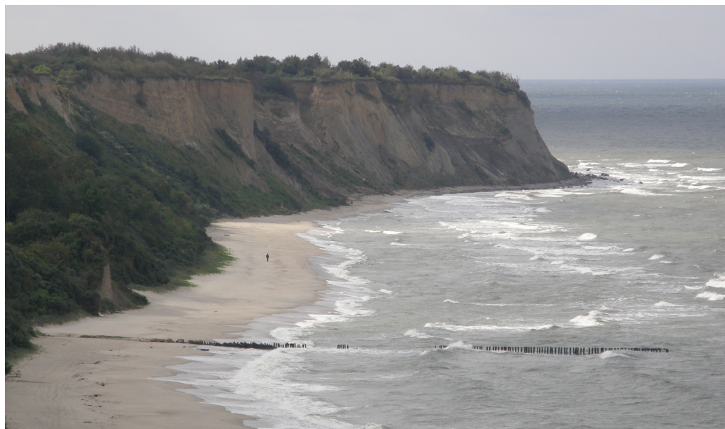
Fig. 6. The single groin near Donskoye (northern part of the western coast of the Sambia Peninsula) constructed in 1938 for protection of the wastewater pipeline outlet
