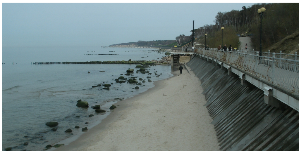
Fig. 9. A massive permeable revetment with pavement on top in Pionerskiy, built in 2008 (570 m long) and extended by 1 km eastwards in 2011
