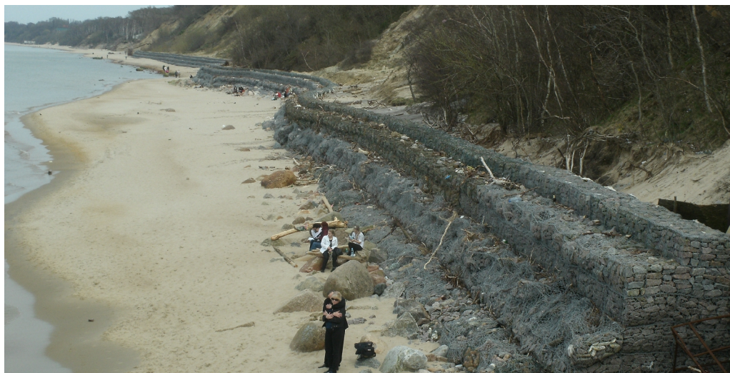
Fig. 8. Gabion structures near Svetlogorsk built in 2009
