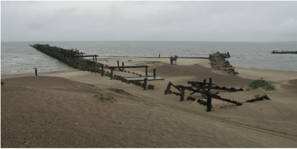
Fig. 14. Old harbour breakwaters in Sventoji, built in the 1920s and 1930s
