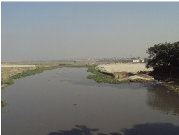
Fig. 16 – Land filling shrinks the canal.
