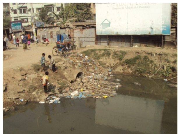
Fig. 9 – A narrow pipe beneath the road allows canal flow.
