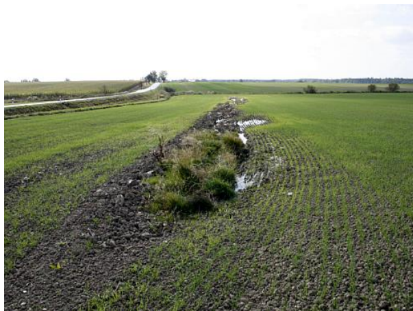
Photos 1, 2 – Examples of drainage system malfunctions – drainage water emergence with the water erosion caused. Source: Z. Kulavý, M. Čmelík – RISWC
