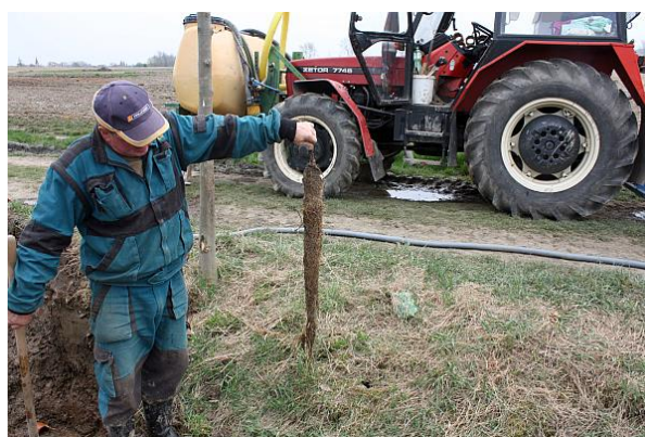
Photos 3, 4 – Examples of drainage system malfunctions – footstalks and roots in the pipes. Source: M. Čmelík – RISWC
