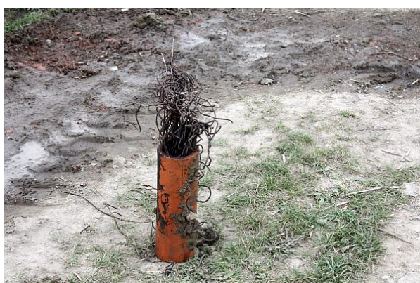
Photos 3, 4 – Examples of drainage system malfunctions – footstalks and roots in the pipes. Source: M. Čmelík – RISWC
