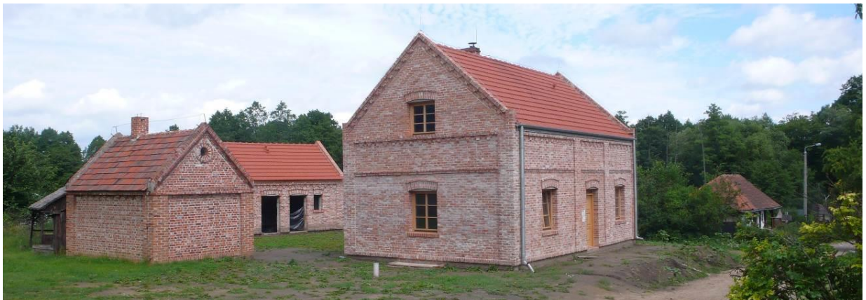
Fig 7. Kujawsko - Dobrzyński Ethnographic Park in Kłóbka, new museum education and cultural centre under construction (reconstruction of traditional rural settling). Photo: Anna Pawlikowska-Piechotka (2014)
