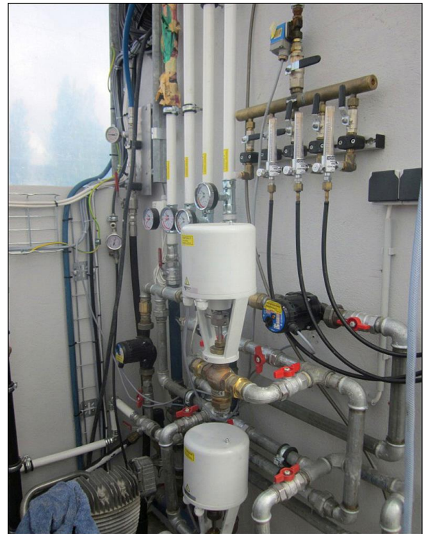
Fig 4. An example of a computerized system in a geothermal greenhouse in Iceland. This system automatically controls temperature, water, fertilizer, and a variety of other growing factors. (Photos by Author)
