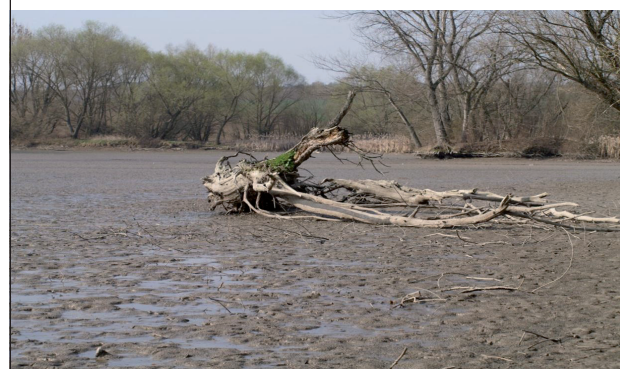
Figure 2: Reservoir filled by sediments. Photo: Jurik, 2017
