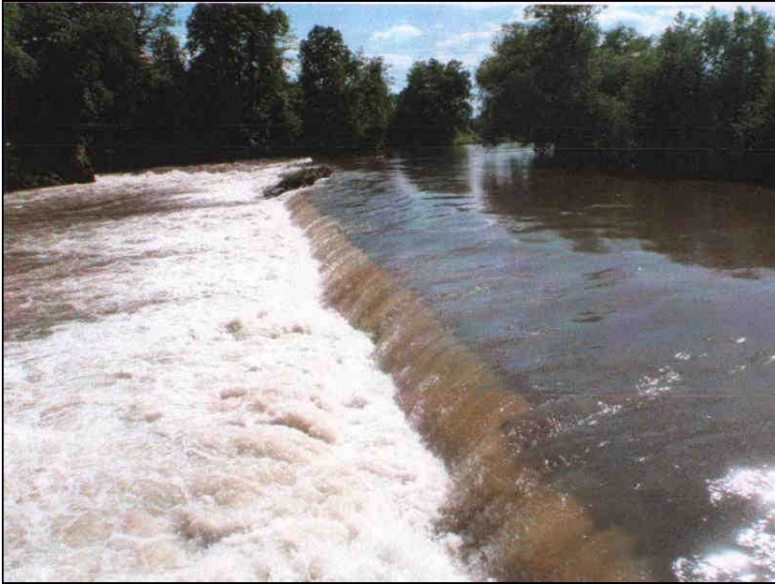
Fig. 2. One of the eight locations selected for a possible small hydropower plant: the Nysa Klodzka River at km 98.74
