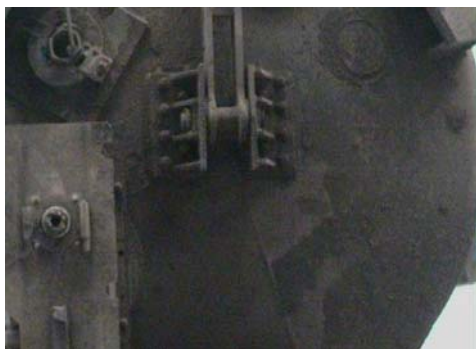
Fig. 17. Metallurgical steel ladle 3
