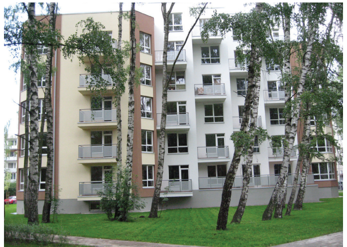
Fig. 5. Infill development with no extra appropriation of open space in Progresā 3 [Photo: S.Treija].
