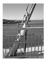
Fig. 5. Cable vibration dampers based on MR fluid technology (https://www.dywidag-systems.com/emea/projects/projectdetails/article/dr-franjo-tudjmann-bridge-dubrovnik-croatia.html)
