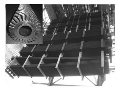
Fig. 2. Heat exchangers constructed of finned tubes used in gas boilers
