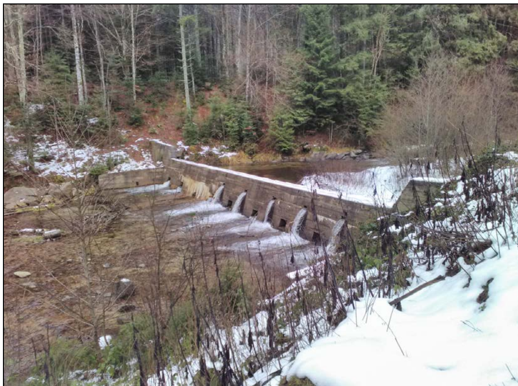
Figure 4b: The discharge sill on the tributary of the Bistra River.
