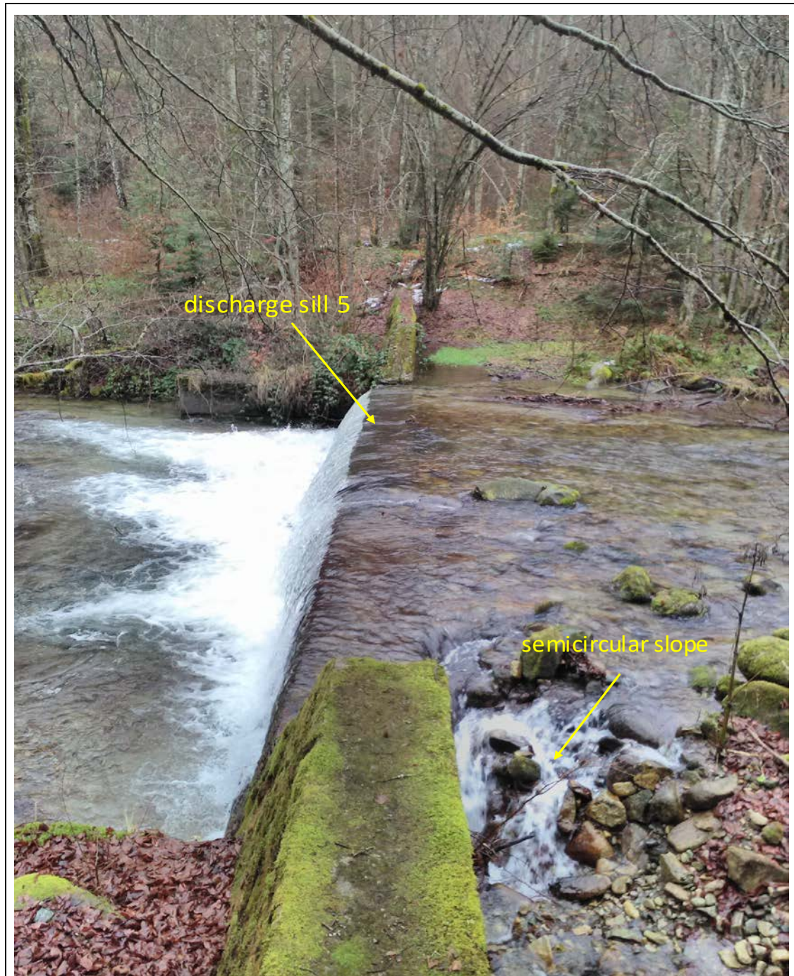
Figure 12: Capturing water in the existing breach with the help of the semicircular slope.
