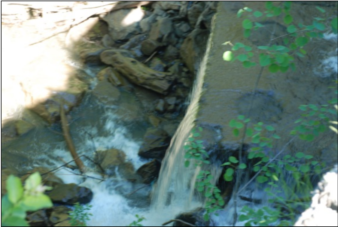
Figure 6: Concrete threshold of three m height, with no fish ladder on the upper Vișeu River.
