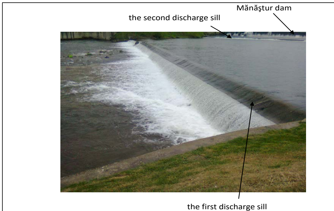
Figure 3: The first discharge sill downstream of Mănăştur dam.
