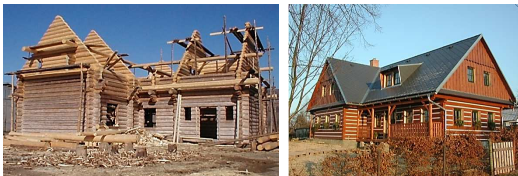
Figure 1: Log construction system [12], [13]
