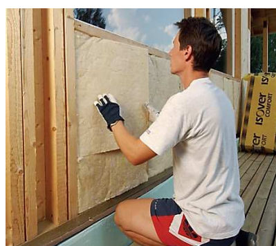
Figure 3: Inserting thermal insulation of walls [17]
