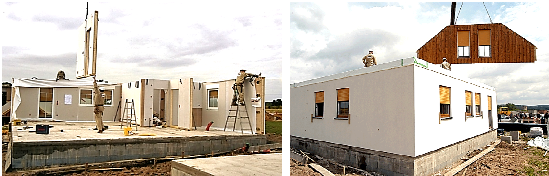
Figure 5: Construction of panel construction system [19]
