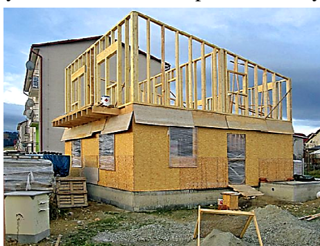
Figure 2: Wooden frame system [17]
