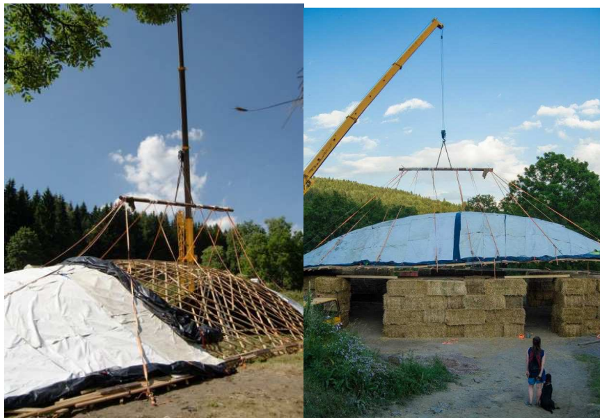
Figure 15: Roof covering with canvas Figure 16: Finished roof placing
