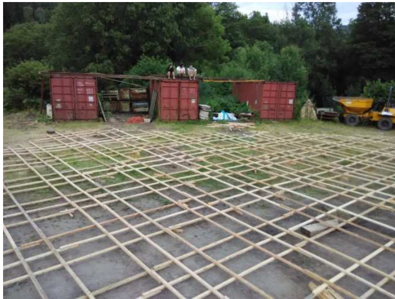
Figure 13: - Flat grid mesh before erection
