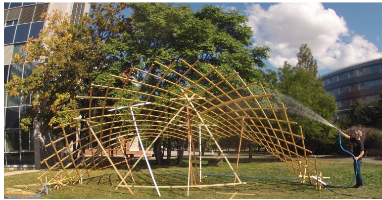
Figure 10: Erection procedure – final shape supported and anchored
