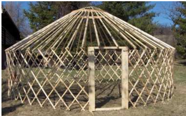
Figure 1: Mongolian Yurt – structural solution
