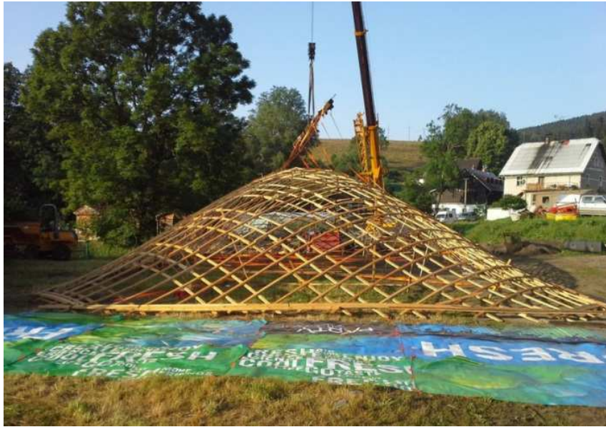
Figure 14: Erected Grid mesh, peripheral fixation
