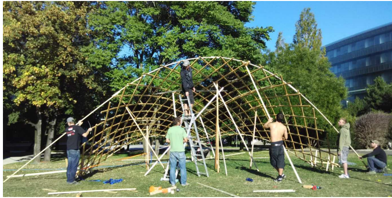
Figure 11: Final shape perimeter tightening
