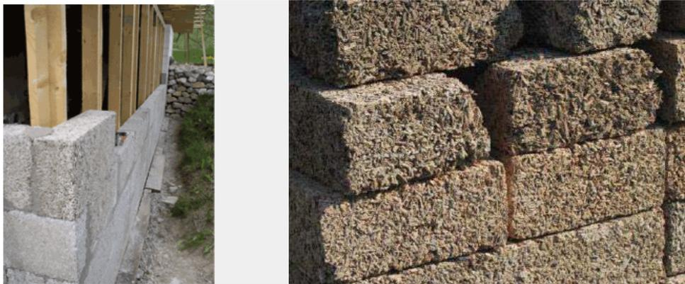
Figure 2: Thermal insulation by Hempcrete panels and prefabricated Hempcrete panels [10]
