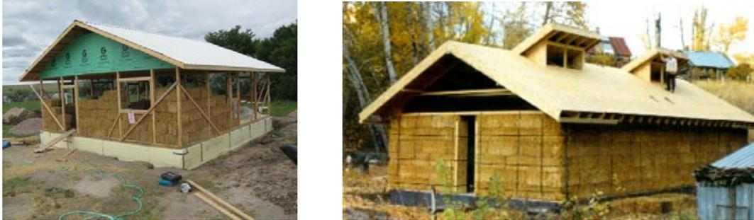
Figure 3: Straw bale as a non load-bearing construction and load-bearing construction (system Nebraska) [13]
