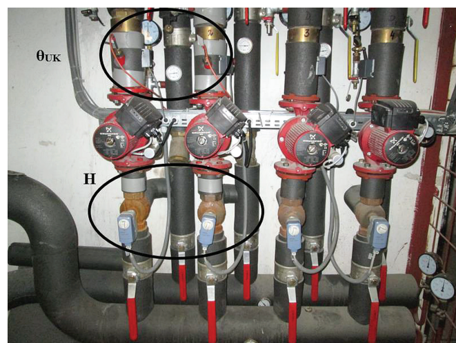
Fig. 4 Location of heat sensors in the room with the heat source \theta_{UK} - supply water temperature - branch V1 (north-eastern) and branch V2 (south-western), H stroke of three-way control valves
