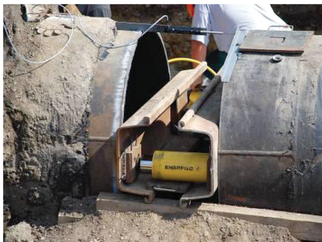
Fig. 22 The loading from hydraulic presses
