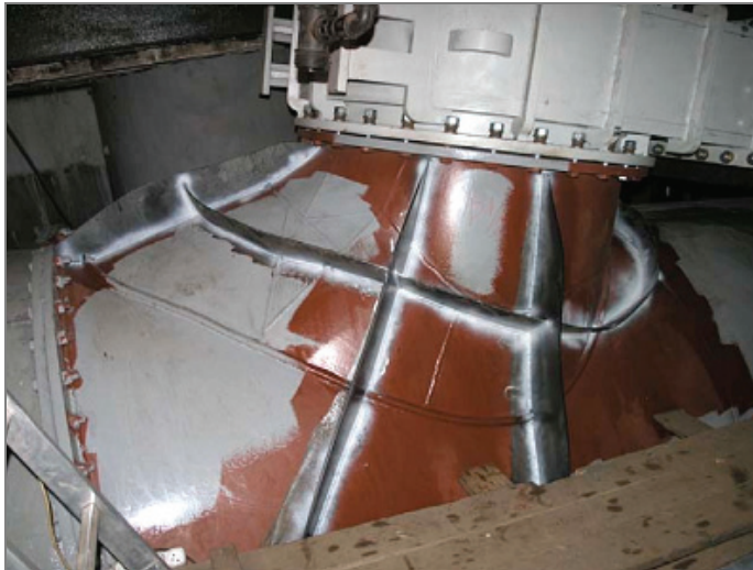
Fig. 19. Bracing webs with reinforcement ring on the inlet pipe. Source: prepared by the authors
