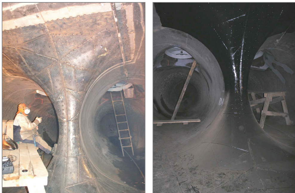
Fig. 17. Structure welding of the reinforcement components to the coating of the pipeline branch and the completed painted plating of the pipeline branch.
