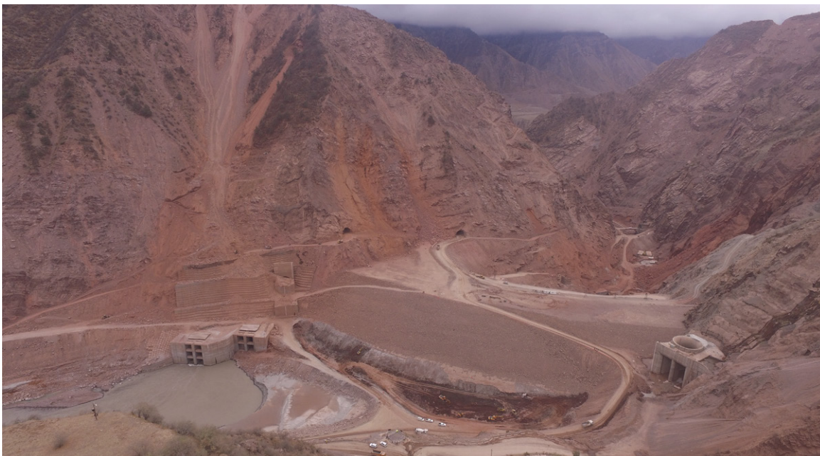
Figure 1: A view on existing cofferdam (50 m high), valley to be filled and underground structures in the hydropower project of a future main dam (330 m high).
