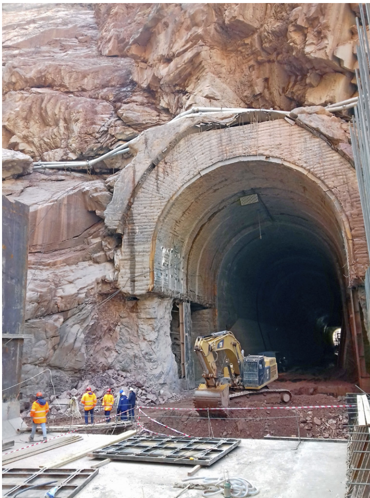
Figure 2 (a and b): Waterway tunnel portals and foundation construction of connection tunnels.
