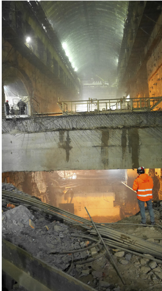
Figure 7: Powerhouse cavern under excavation of lower part.
