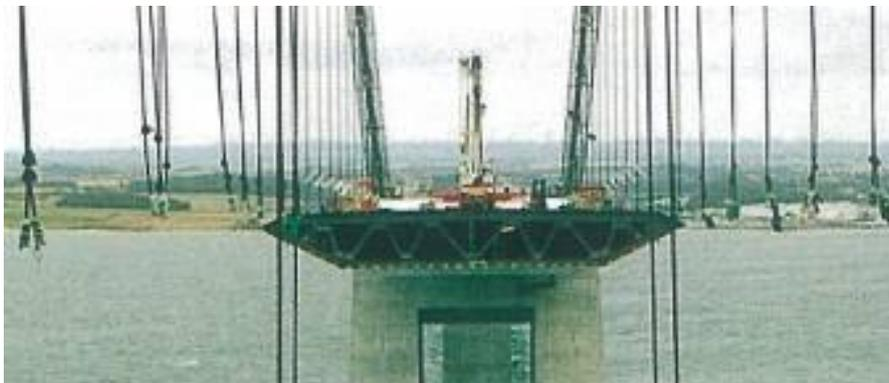
**Figure 8.** Storebaelt Bridge deck (1998), depth ~ 4.5 m, self weight ~ 0.35 t/m<sup>2</sup>
