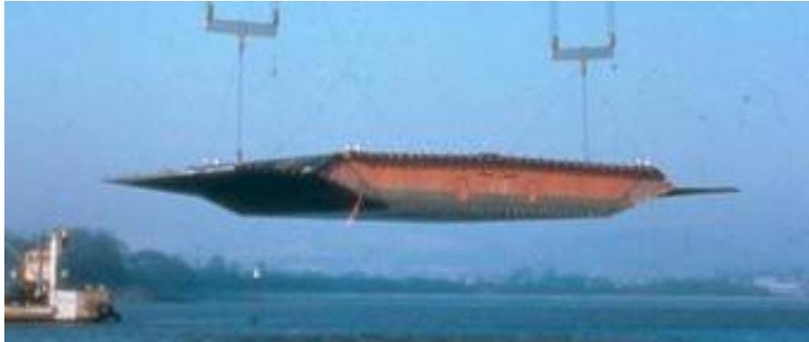
**Figure 7.** Severn Bridge deck (1966), depth ~ 3 m, self weight ~ 0.3 t/m<sup>2</sup>
