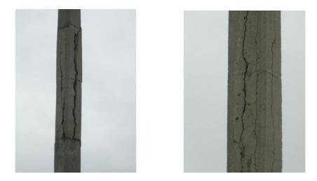
Figure 2. Cracks at some of the bridge concrete hangers
