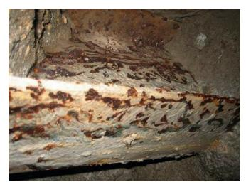
Fig. 8. Steel corrosion in primary support of subsea tunnel
