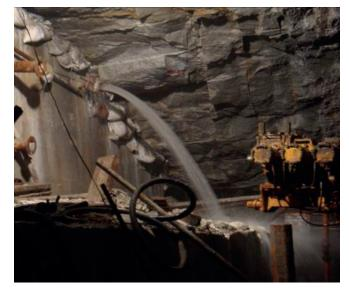
(a) Large amount of water in tunnel before grouting
