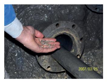
(b) Tunnel water disappeared after grouting Fig.7. Grouting and water plugging at whole cross-section of F1 weathered trough
