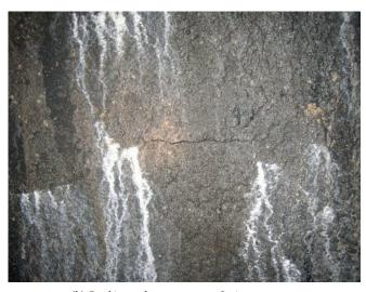
(b) Cracking and water seepage of primary support Fig.6. Schematic diagram of cracking and water seepage of primary support on site
