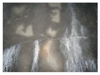
(a) Cracking and water seepage of primary support
