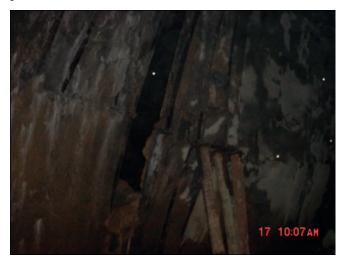
*Fig. 4. Concrete peeling and steel arch distortion of primary support in subsea tunnels*
