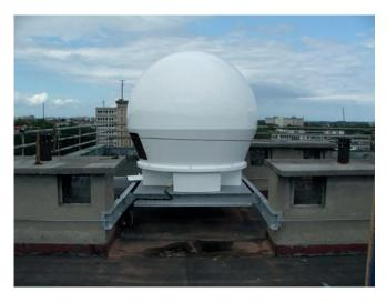
Fig. 1a. 1.5 metre HRPT-MetOp antenna in radome
